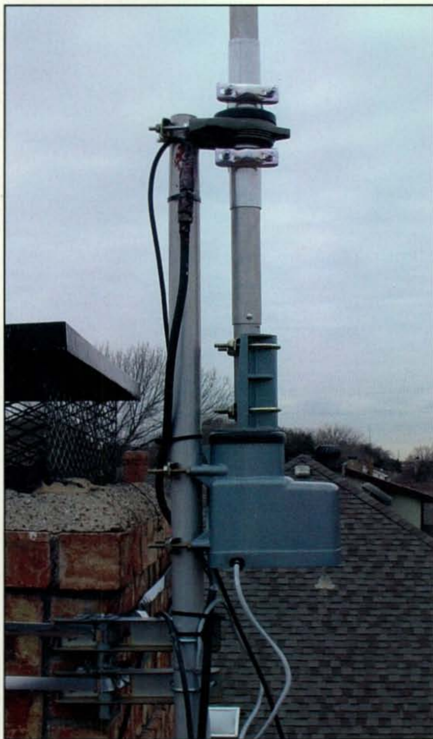
Photo A— The TB-105 and AR-35 mounted on the author's chimney. The TB-105 is at the very top of the lower mast section.
